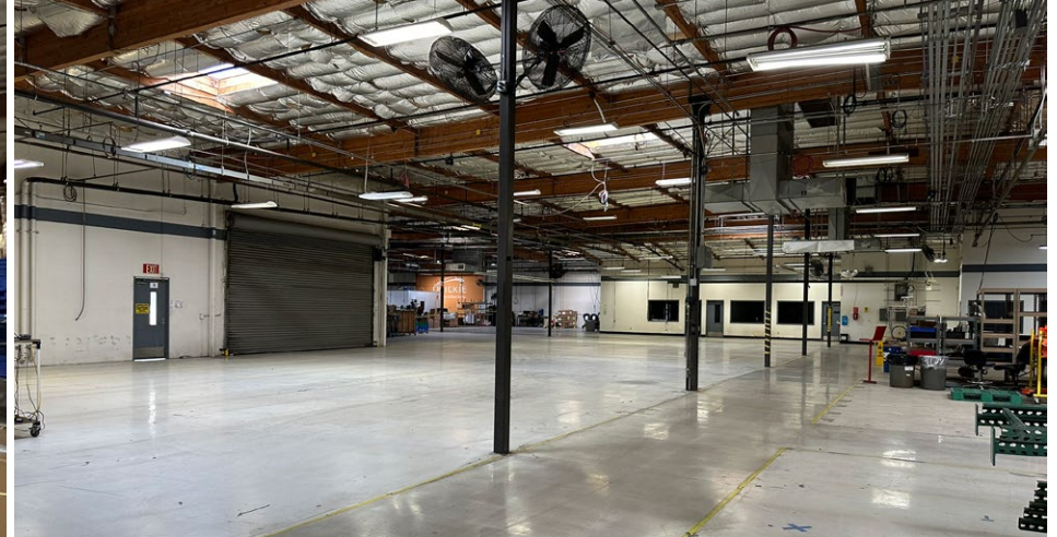
MANUFACTURING OR WAREHOUSE
