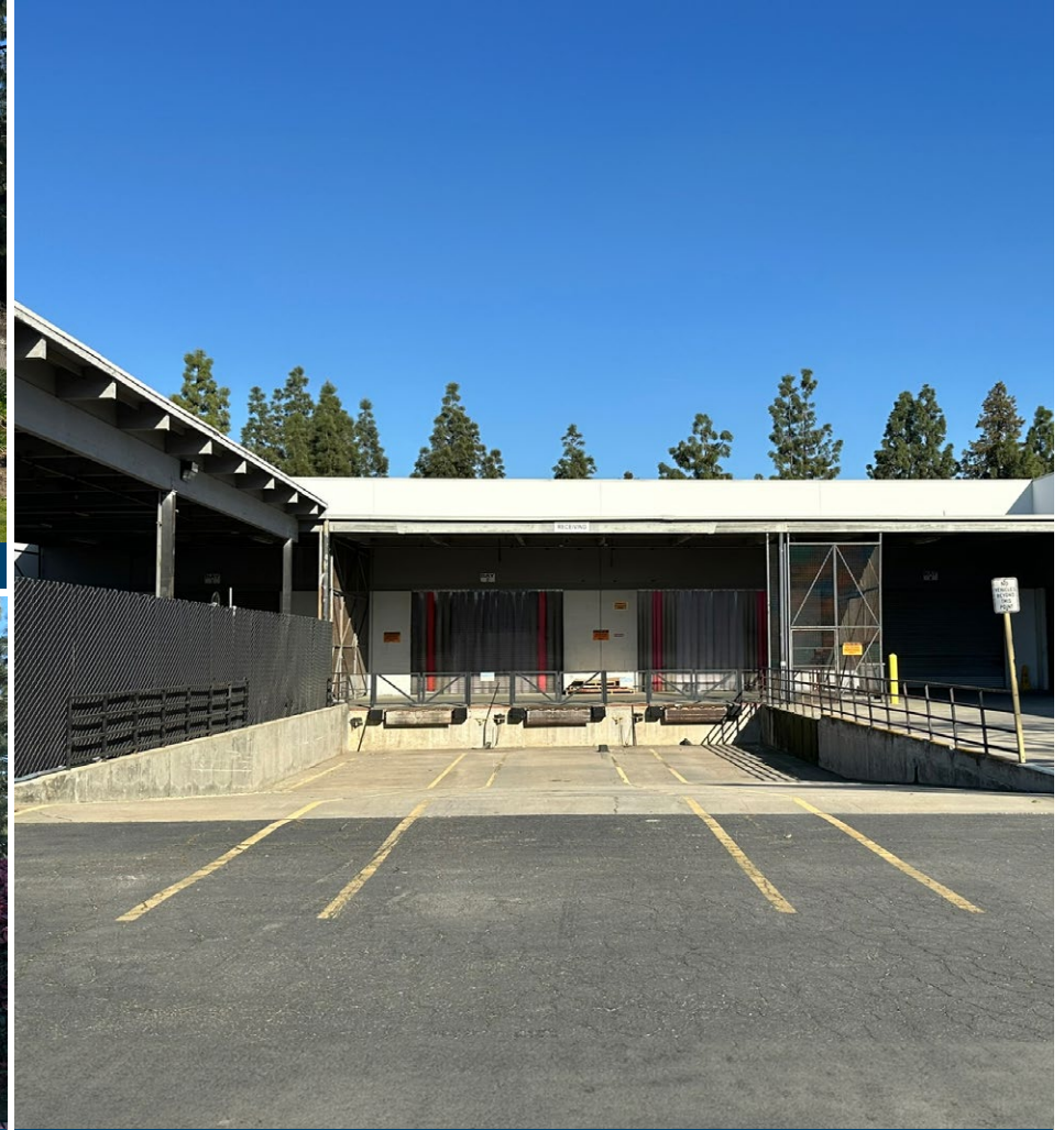
TYPICAL LOADING DOCK
