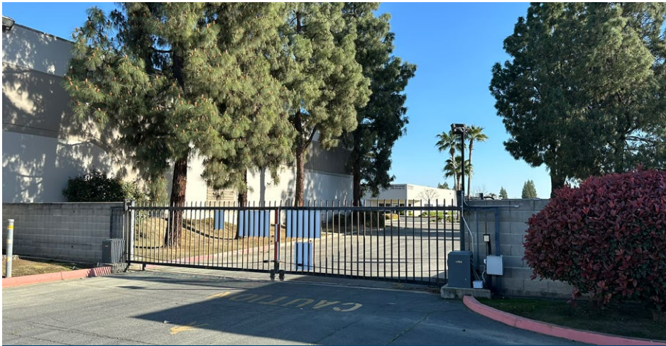
AUTOMATIC CONTROL ACCESS GATE TO INTERIOR LOADING AREA
